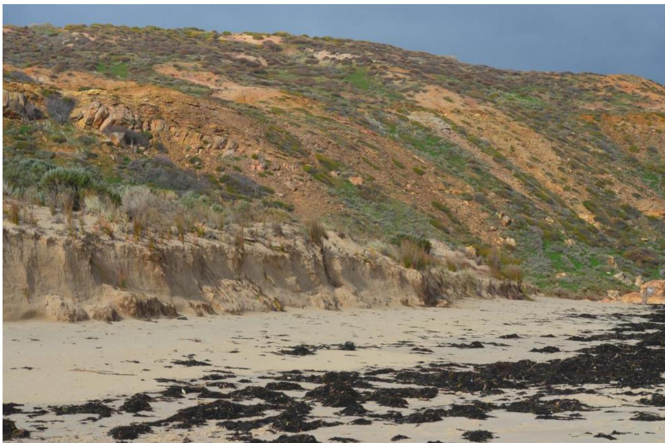
Image 27. Foredune erosion following winter storm events, June 2025 Ochre Cove (Photo: S & A Read)
